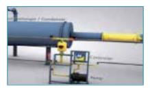
A PLC controlled pump forces water through the piping loop. Once the water enters the Pod Storage Unit, the system periodically injects the cleaning pods into the inlet pipe. Following injection, normal system water flow carries the pods through the inlet pipe and into the main line.
